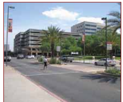
Pedestrian crossing treatment designed for pedestrian and bicycle access and safety.
