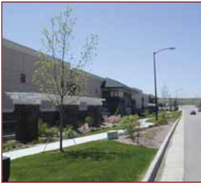
Equal attention shall be paid to all sides of a building, as illustrated on the back of this commercial center which adjoins a residential area.
