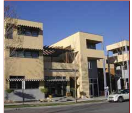
Live-work units within a mixed-use activity center incorporate professional offices at the street level and residences above.
