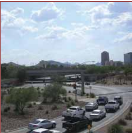
Continuous pedestrian and bicycle facilities were successfully provided through this busy intersection.
