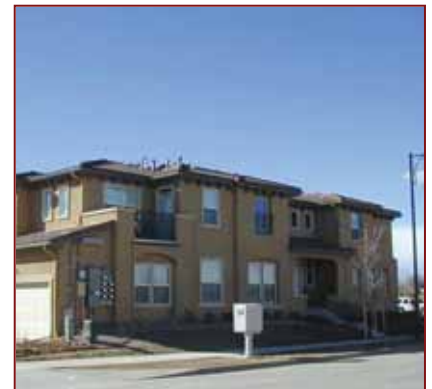
The massing and use of exterior materials on multi-family buildings of ten units or less shall be arranged to give each building the appearance of a large single family home.
