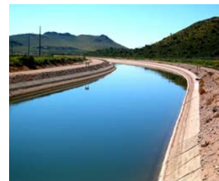
CAP distribution line
