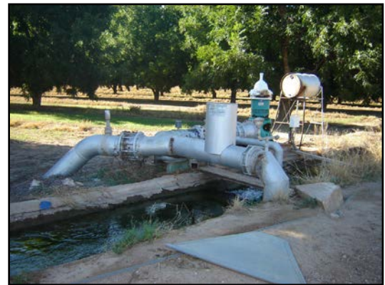
Existing groundwater well
