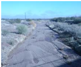
Sahuarita Road looking south
