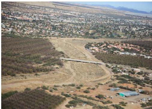
Continental Bridge looking north
