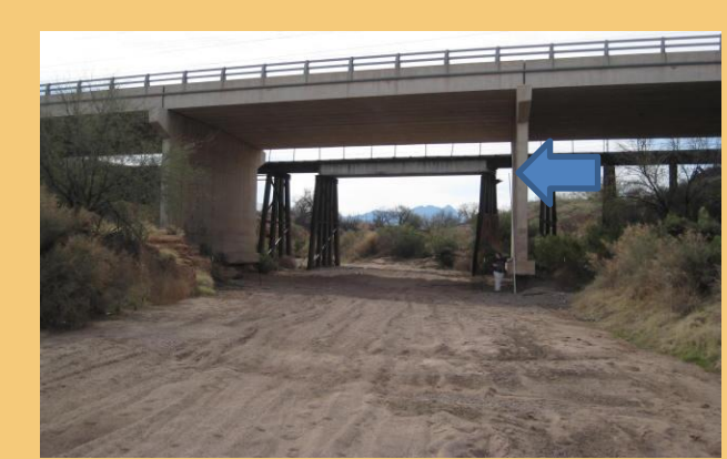
Photo # 8. Looking upstream at Pima Mine Road Bridge The arrow points at the top of a 16 ft. survey rod.
