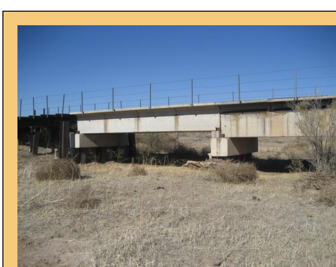
Photo #15. UPRR Spur bridge. This picture shows two segments of the bridge. The bridge was destroyed during the 1993 flood.
