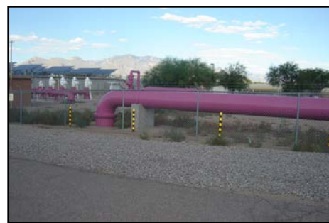
Purple irrigation pipes for treated effluent
